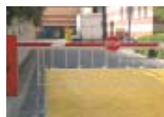
Barrier Relay Control Page 95
